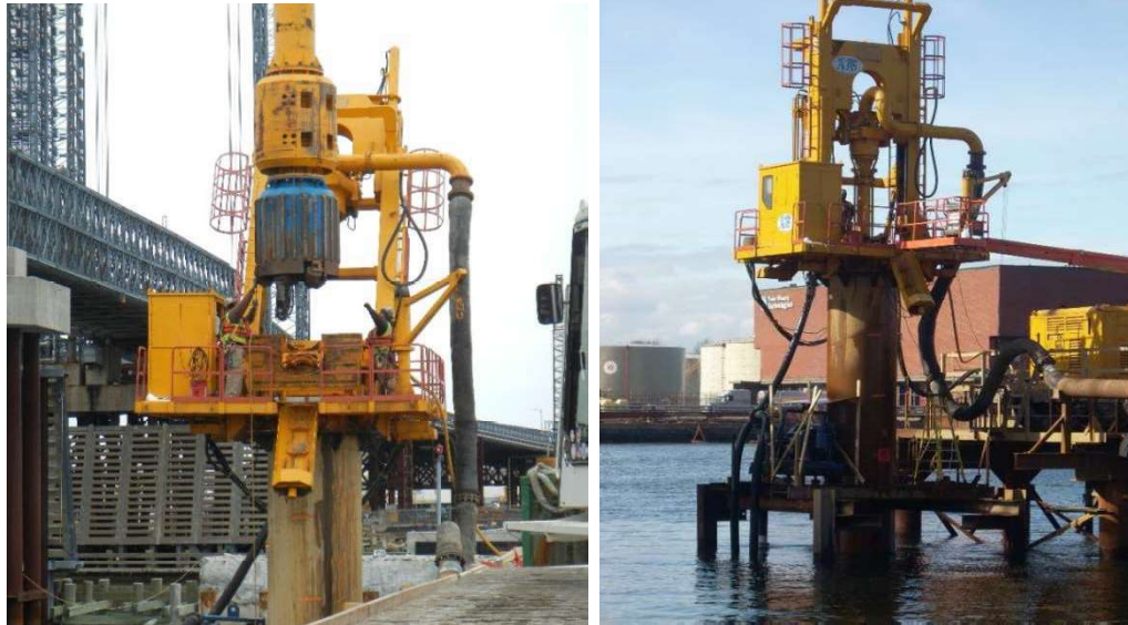
Figure 4-10 Top-Drive Reverse Circulation Drill
