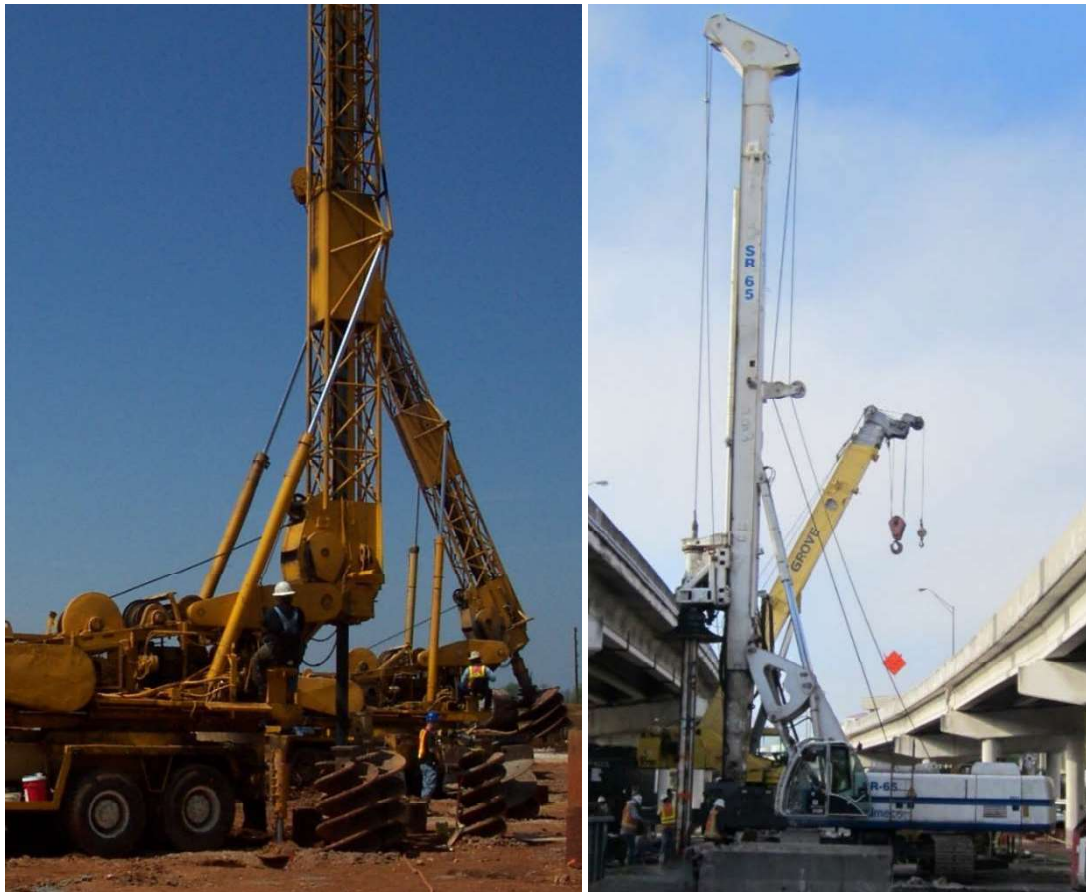
Figure 4-3 Mechanical (left) and Hydraulic (right) Powered Drilling Machines
