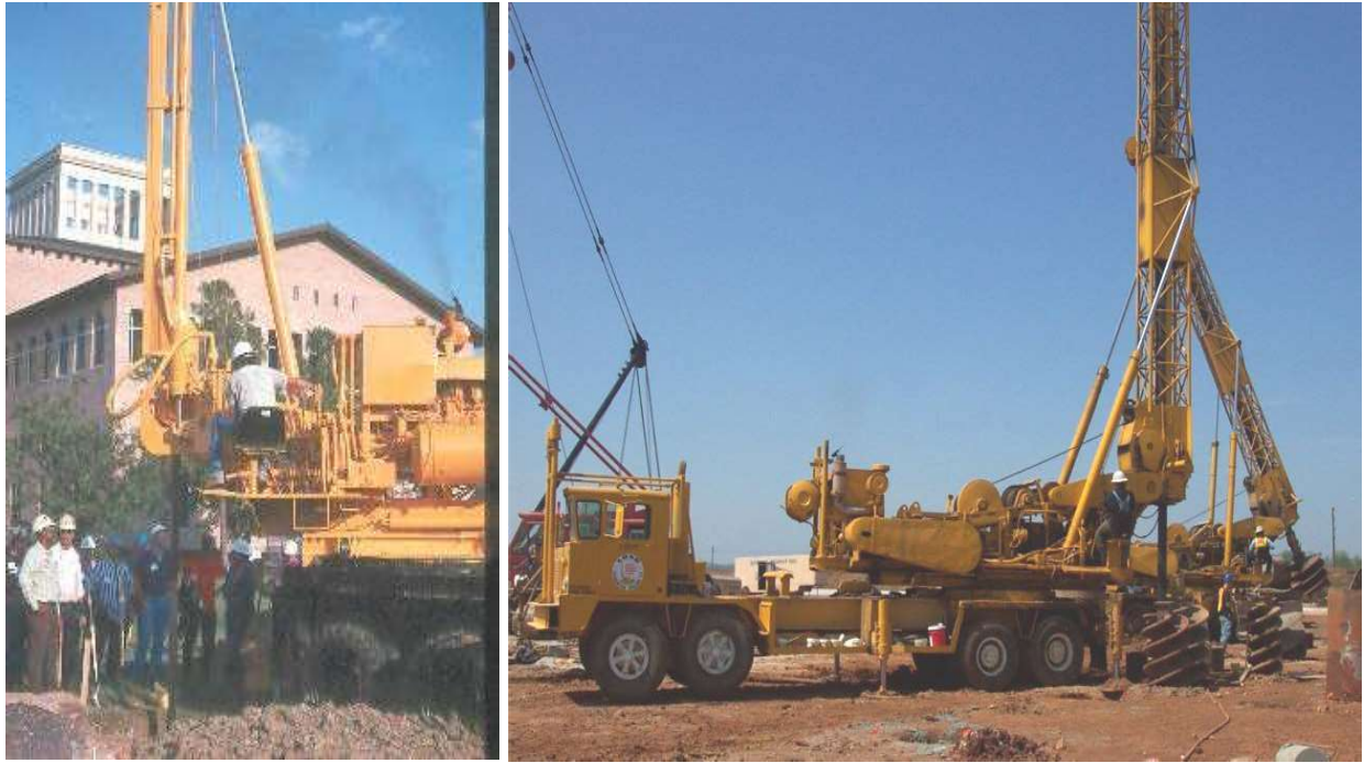
Figure 4-4 Truck Mounted Drilling Rigs
