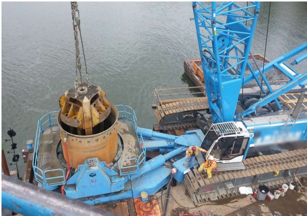
Figure 4-8 Oscillator Machine
