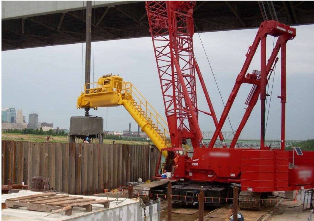
Figure 4-5 Crane Mounted Drilling Rig
