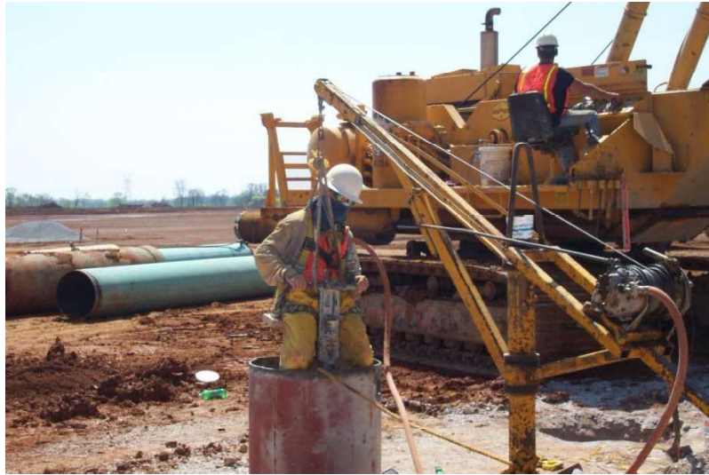
Figure 4-12 Manual Excavation in Rock
