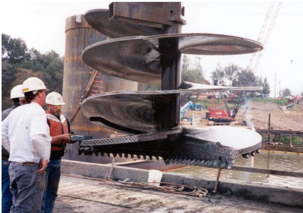
Figure 4-17 Large Diameter Auger with Double Cutting Edge
