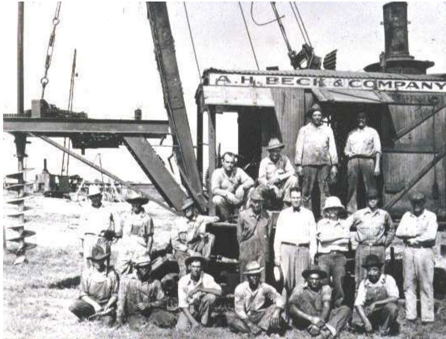
Figure 4-1 An Early Drilled Shaft Machine and Crew
