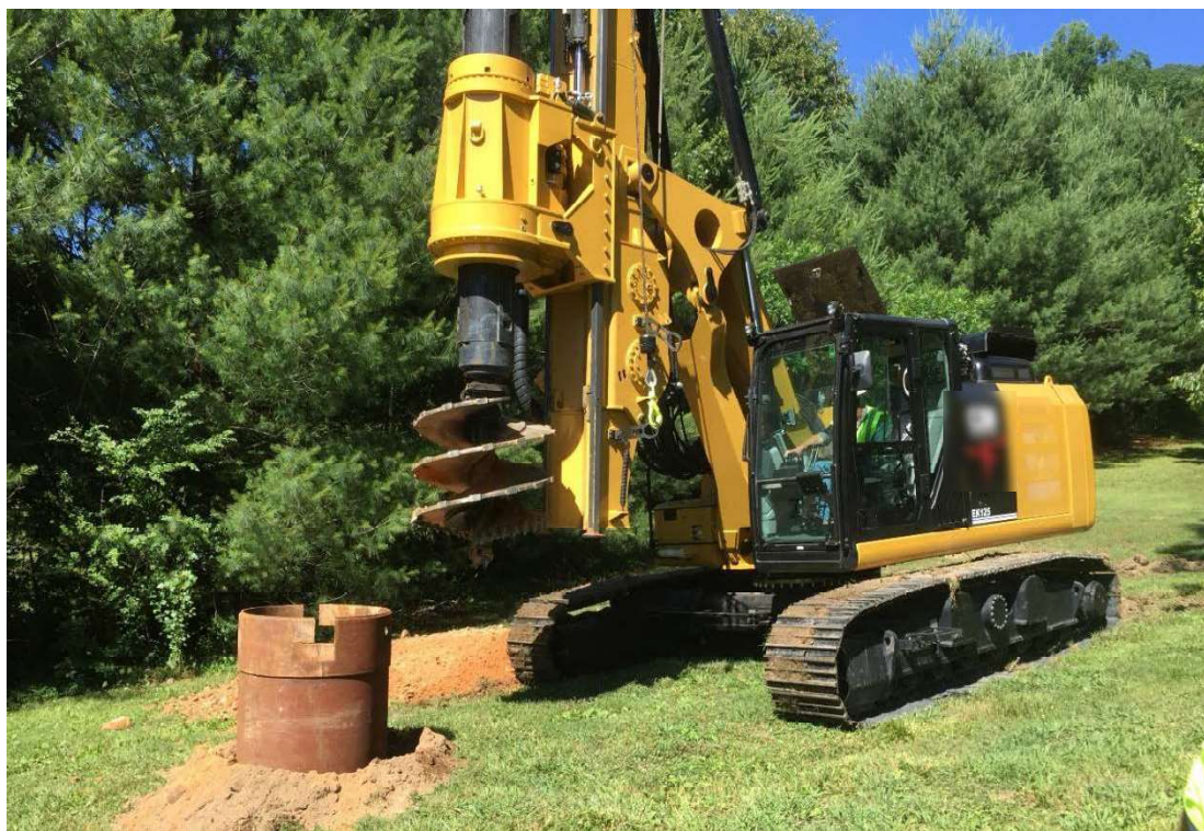
Figure 4-6 Crawler Mounted Drilling Rig
