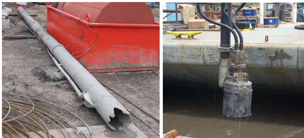
Figure 4-33 Airlift and Hydraulic Pumps for Shaft Base Cleanout
